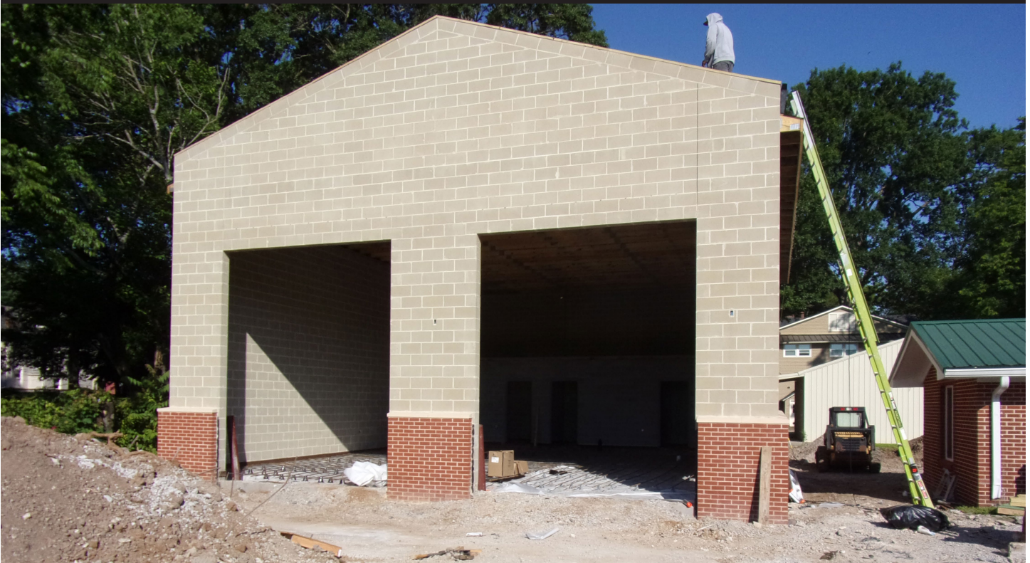
New Fire Station Bay under construction on Bond Street.
