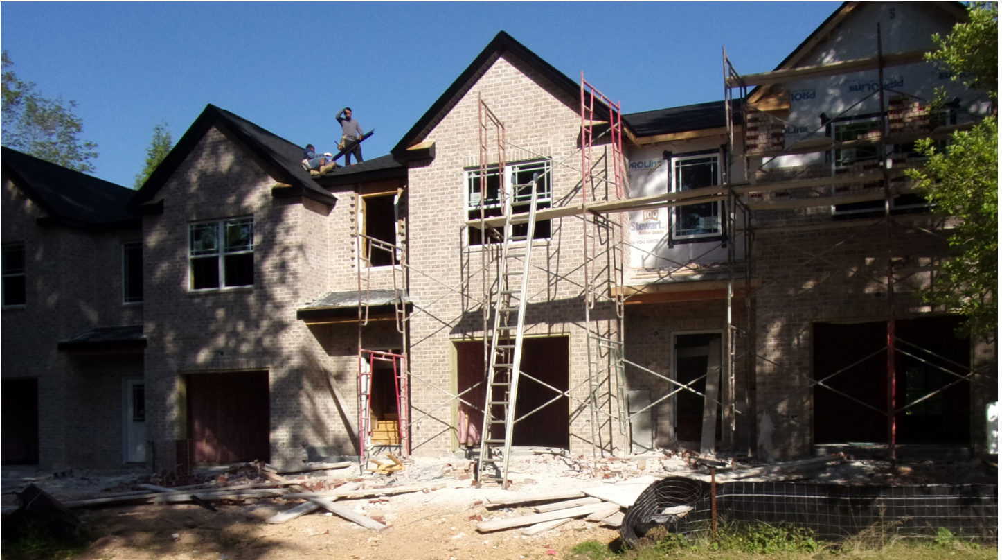
New Townhomes being built on South Walnut Street.
