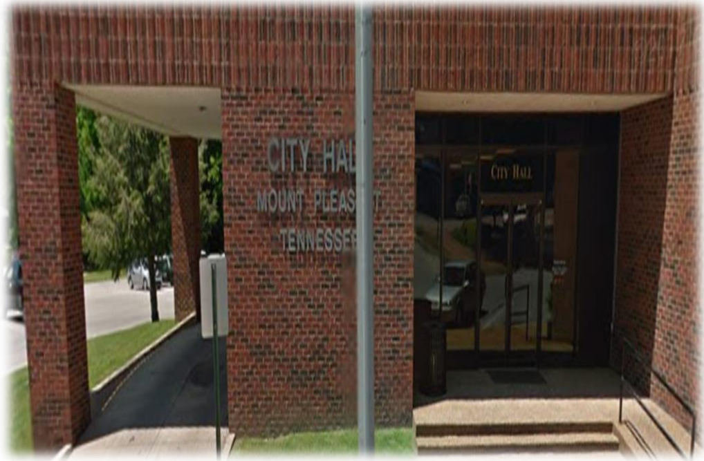
Integration of ramps and stairs allows access for everyone.
