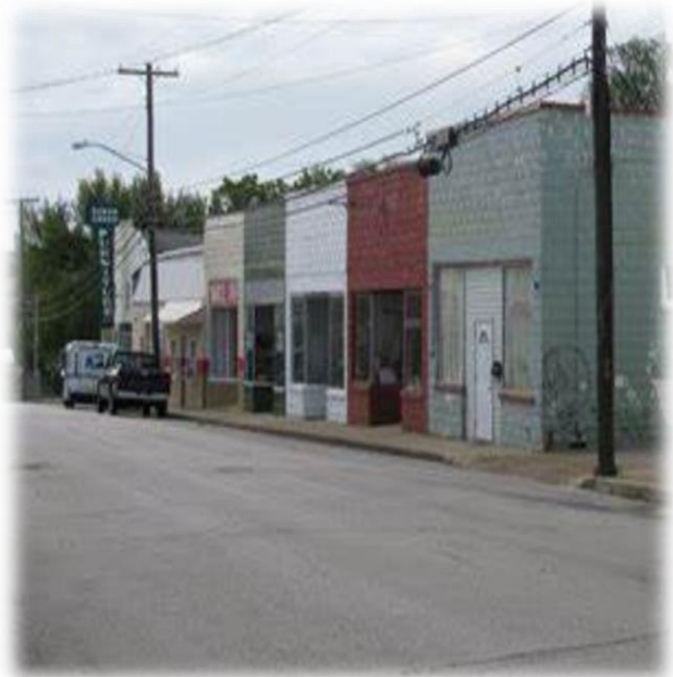
The repainting of a brick building should be done carefully and thoroughly.
