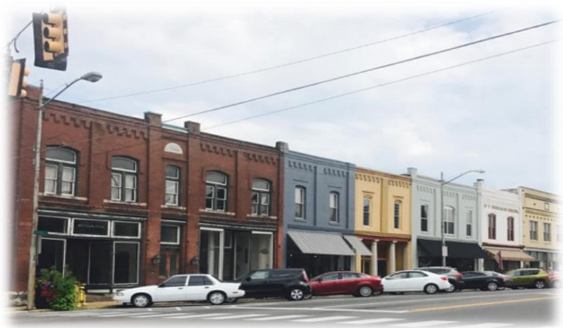
Mount Pleasant has a variety of original and retrofitted storefronts.
