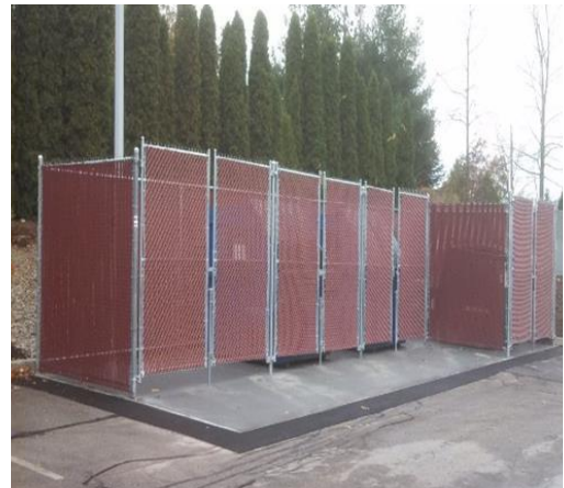
Inappropriately screened garbage collection areas
