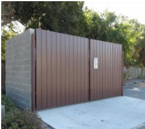
Appropriately screened garbage collection areas
