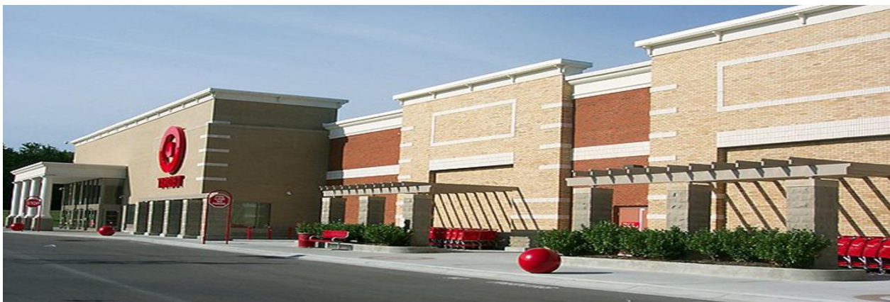
Screening of grocery cart storage
