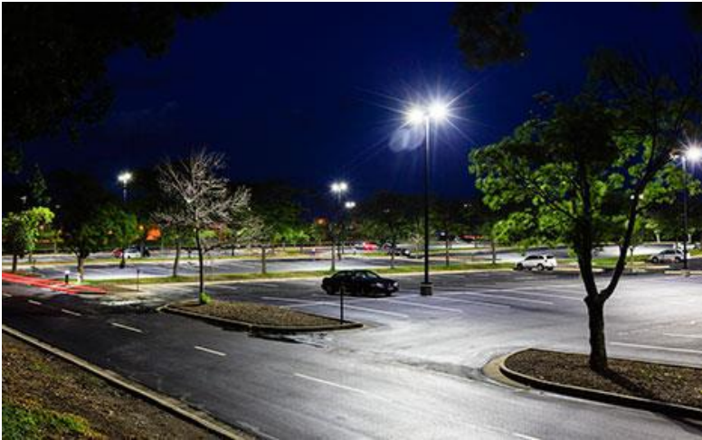
Parking lot lighting (low intensity)
